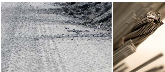
Milling debris/construction sites
